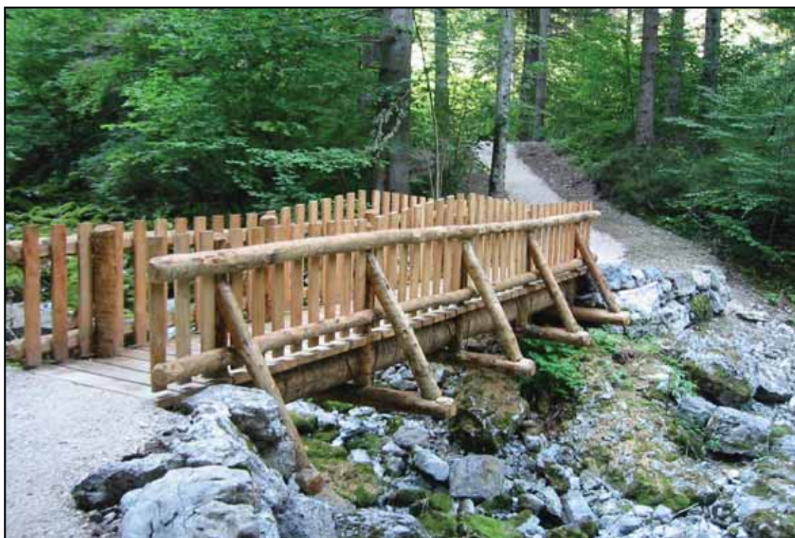
Stretch of footpath equipped by PNAB for tourist purposes, using local materials
